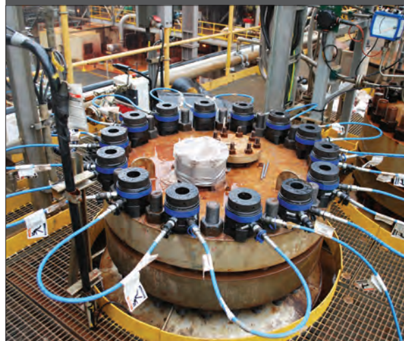
▲ Custom tensioners used for tensioning multiple bolts on pipe line flange
